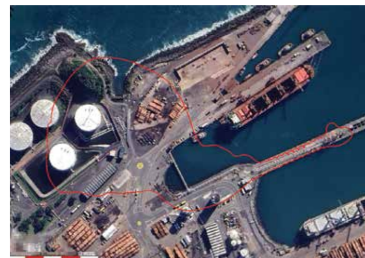
Port Methanol Tank Farm
