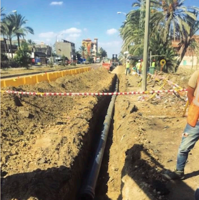
A portion of the pipeline installed to direct plant effluent to community irrigation
