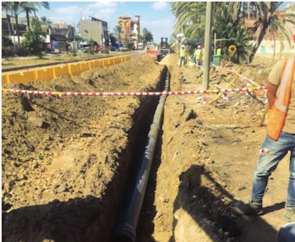
A portion of the pipeline installed to direct plant effluent to community irrigation
