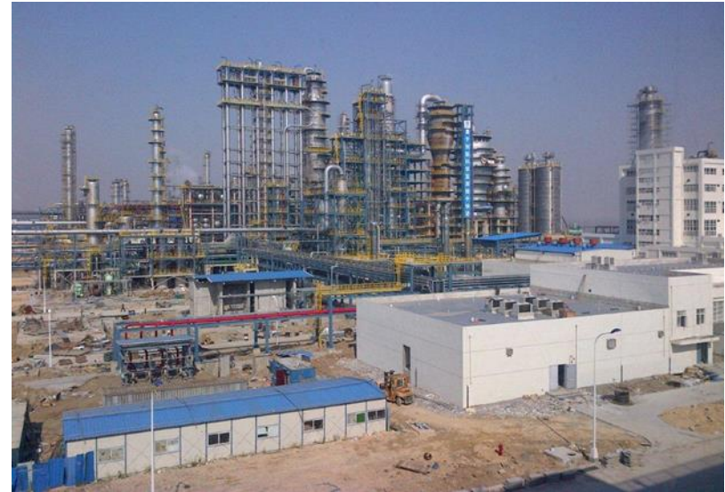
Ningbo Skyford's 1.8 MMT merchant methanol to 0.6 MMT olefins plant
