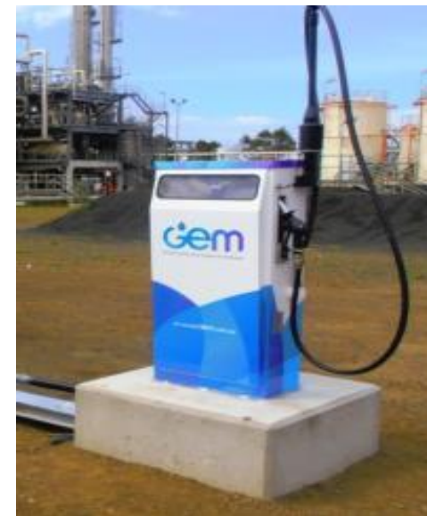
Methanol / gasoline pump at Coogee plant site
