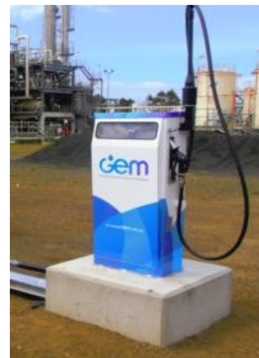
Methanol / gasoline pump at Coogee plant site
