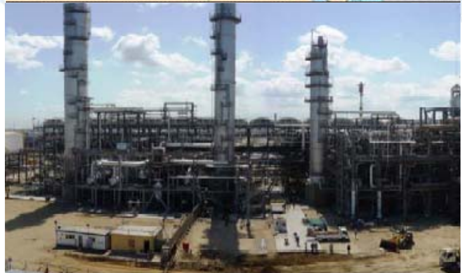
EMethanex Plant Site, March 2010, Mubarak Gas and Petrochemicals Complex, Damietta
